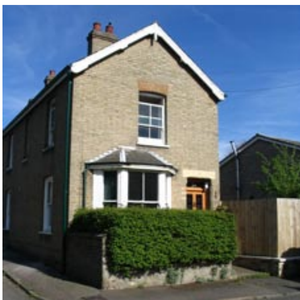
Gable end of No. 34 Black Horse Lane
