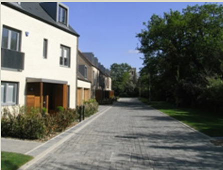
High quality design with minimal 'highway engineering', Trumpington Meadows
