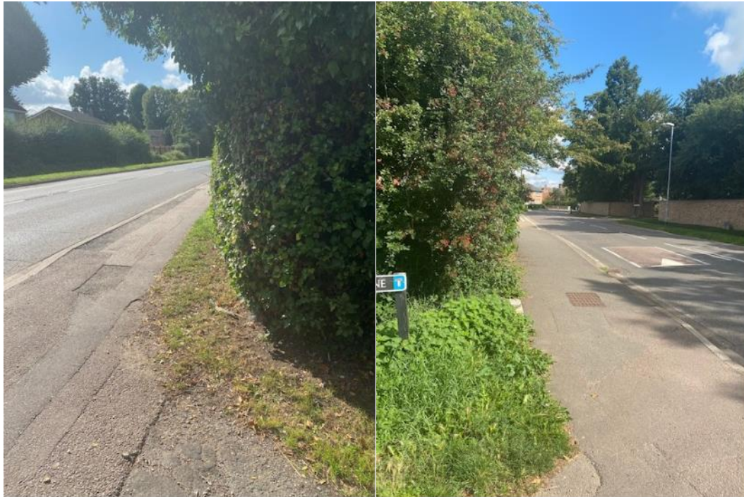
Figure 5 – Fews Lane Junction Visibility 2.4m Set Back Right and Left
