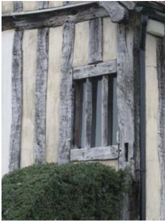
Example of a Mediaeval Diamond mullioned timber
