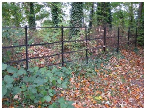
Example of park or estate railings
